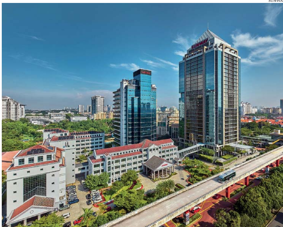
While SunCon benefits from Sunway Bhd's property developments, it is also able to compete against construction heavyweights in securing private and government-led projects, including contracts from MNCs
