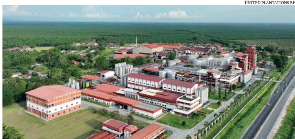
A view of UP's inland refinery, Unitata, which celebrated its golden anniversary after its commissioning in 1974
